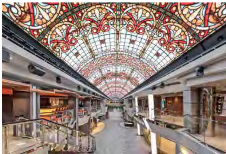
Work in progress: MSC Grandiosa: sister-ship of Meraviglia and Grandiosa - maiden voyage foreseen within end of 2019. MSC Cruise: MUSICA – PREZIOSA – SPLENDIDA - ARMONIA Maintenance of the stage area, curtains and of the movement equipment on stage.
